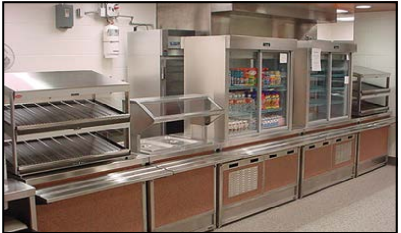
Sturgis High School, Sturgis MI. Consultant: J. Riemenschneider & Associates
