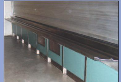
The heart of the Uni-Wall® system is a strong metal stud wall with horizontal utility chase openings for beverage, plumbing and electrical lines - all easily accessible through removeable front panels.
